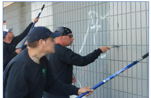
Groundwork PG crew remove graffiti
